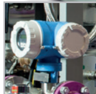
Local instrumentation with either the HART® or the Foundation™ Fieldbus communication protocol
