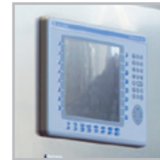
Plant control by a Local Control Panel (LCP) or directly by customer's DCS/ESD
